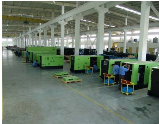
Workshop of silent generator set
